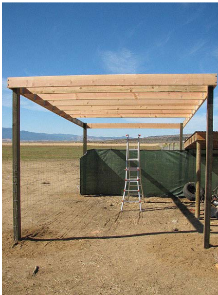
The first trip, the frame was put up.
