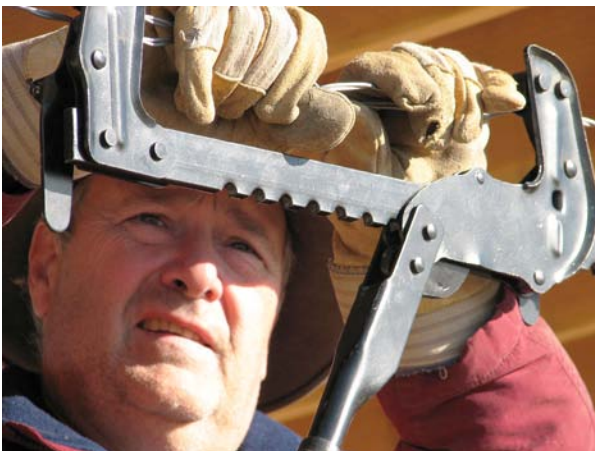
Ken tightens cross wire to reinforce the strength of the frame.
