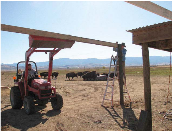
Lenny maneuvers a roofing beam into place for Ken.
