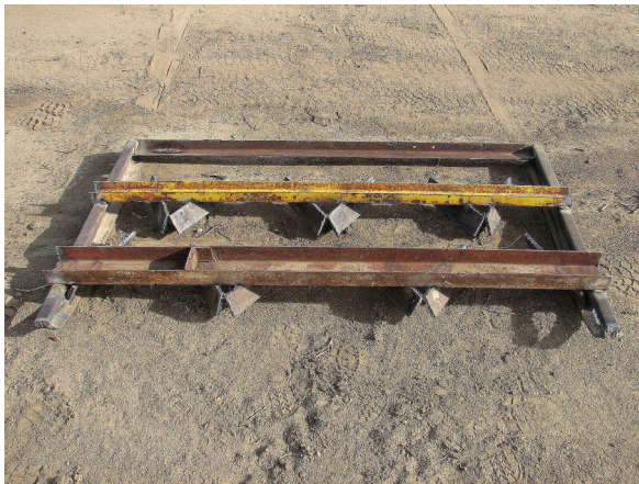
Front view of "above ground plow" used for dragging
